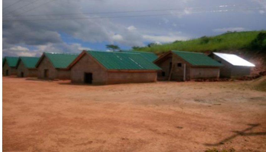
Figure 11: Chalets being constructed by Private Investor Source: Photo taken by Mukuwa (2015)
