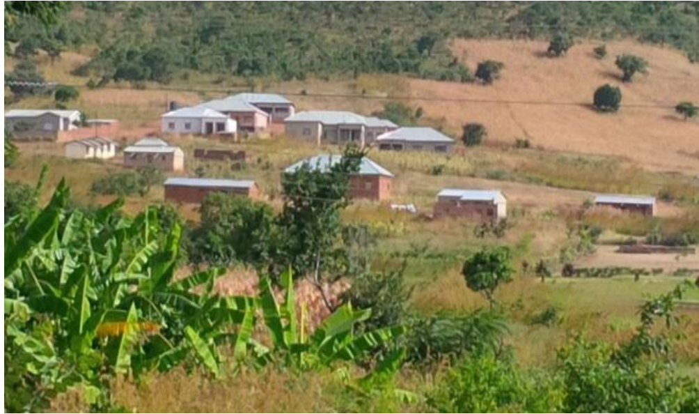
Figure 8: Some Housing development at Mwami Border Source: Photo taken by Mukuwa (2015)
