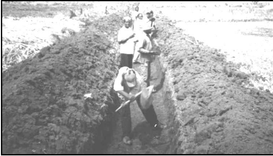
Figure 5: Community participation in pipe line construction (Field work, 2010)
