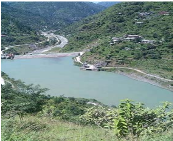
Dam site of Parbati HEP-III: upstream & downstream view
