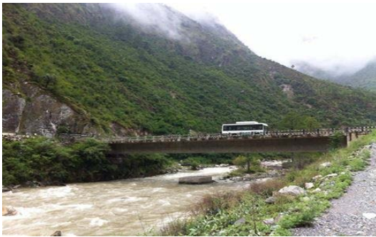
Bridge over River Sainj at Larji village constructed by NHPC Ltd
